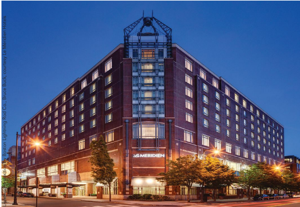
▲ The steel turret atop Le Méridien-MIT Hotel in Cambridge, Mass., acts as a strike-termination device and is connected via the LPS to ground. A conventional air terminal is visible on the parapet in the lower-left corner of the left photo.
