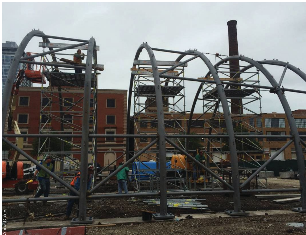
▲ The tube arches were shipped in pairs of two half-arches, with a field splice located at the top of each arch. Up to six arches were assembled at a time on the ground, then lifted into place.
